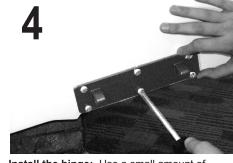
Install the hinge: Use a small amount of marine sealant in each hole. Do not use excessive force when installing screws - ream the hole if necessary. Use a phillips head screw driver to install the screws. Don't use a drill gun.
