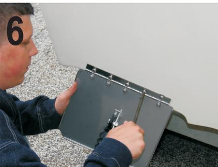
**Attach the Plate:** Using a philip head screw driver attached the plate using the #14x3/4 sheet metal screws that came in bag "A". Do not overtightened these and don't use a screw gun.
